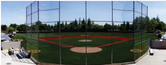
Nick Cecchetti Baseball Field During Final Stages of Renovation
