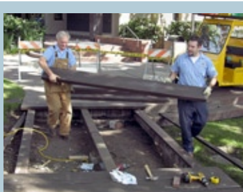
Bruce Michael and Michael Minnema rebuild foot-bridge in center of campus
